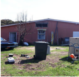
View of: Farm Shed Looking north Inspected on 18.09.2013
