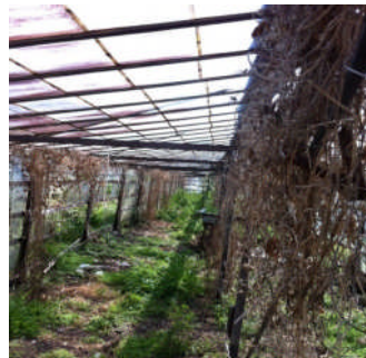
View of: Glass house Inspected on 18.09.2013
