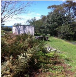
View of: Farm Shed Looking south Inspected on 18.09.2013
